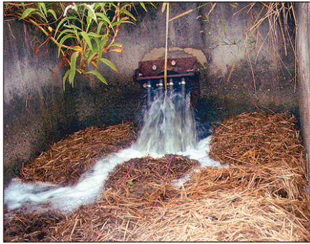
Intake effluent from Merrimac sewerage plant enters Palm Meadows irrigation pond through a trap filled with straw.
